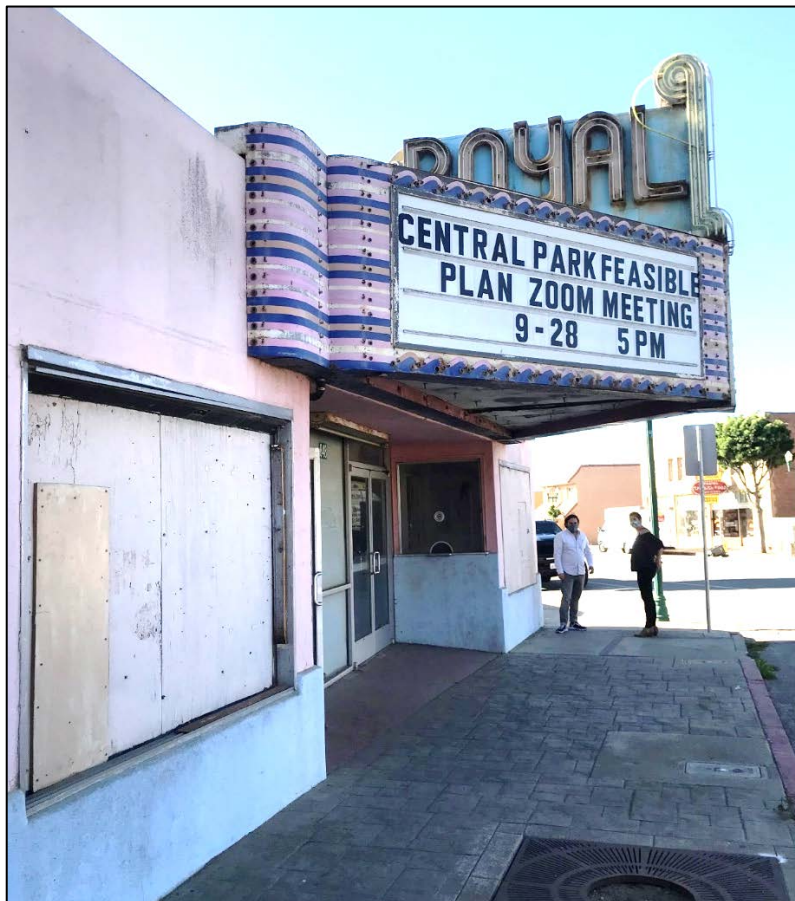
Plate 6. Royal Theater façade, facing south.
