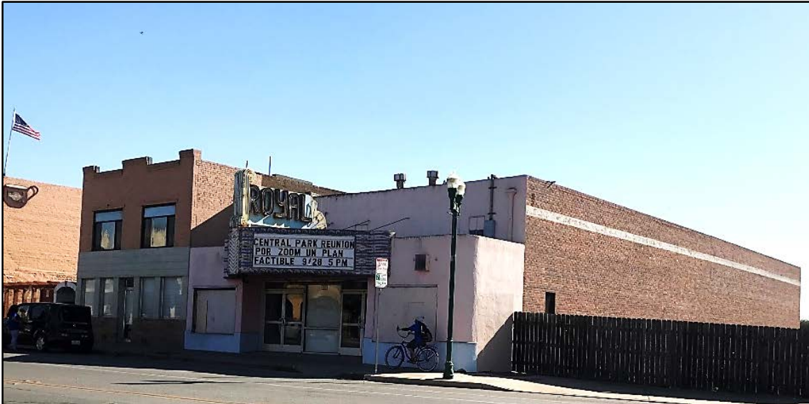
Plate 1. Overview of Royal Theater, facing northeast.
